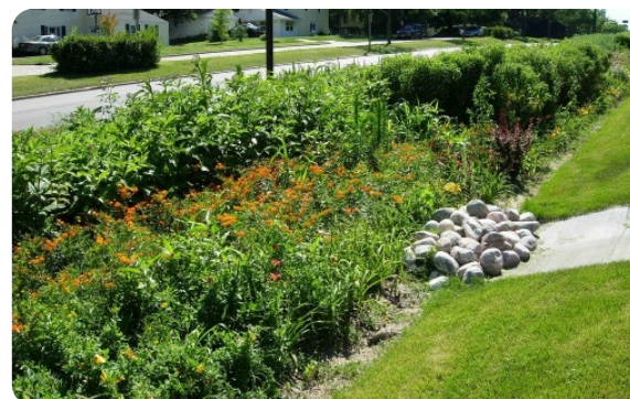
Improvements to grass swale areas can increase stormwater management efficiency, better filtrate rainwater, and add a visually aesthetic appearance.
